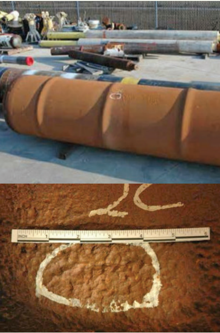
Figure 7 Wrinklebend sample having severe pitting.
