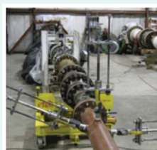
Three Traversing Pitot Tubes Installed Downstream of an 8" Flow Conditioner
