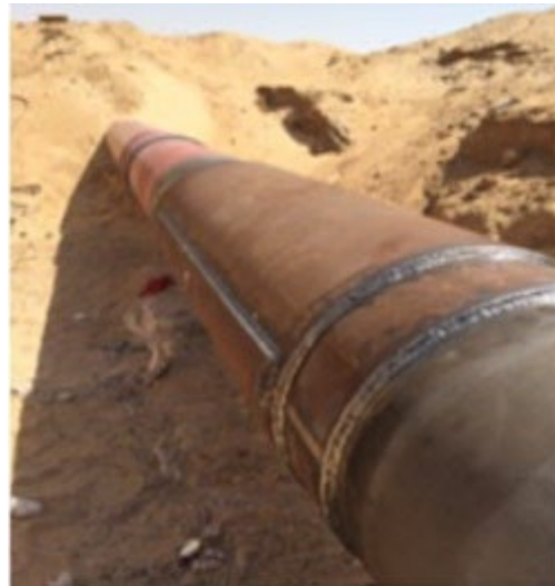
Adjacent tight-fitting sleeves installed
