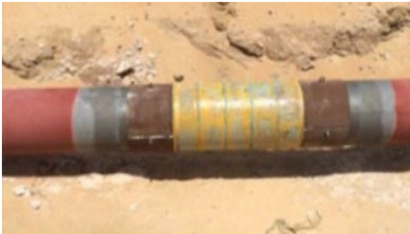
Adjacent tight-fitting sleeves installed
