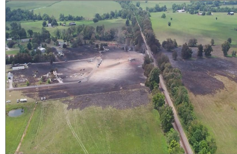
Enbridge near Danville, Kentucky on August 1, 2019 30" x 0.375", X52 A.O. Smith, Flash Welded 1942 Installation (amended CAO)
